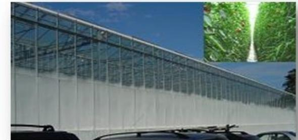
Paint spray for shading
